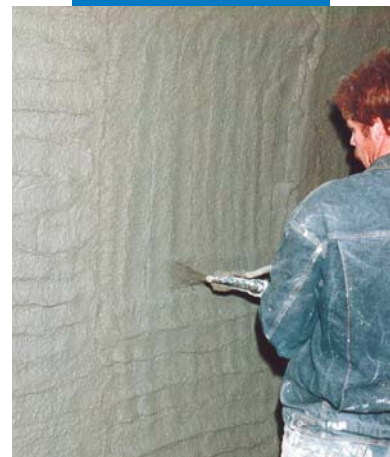
Spray application of Nivoplan
