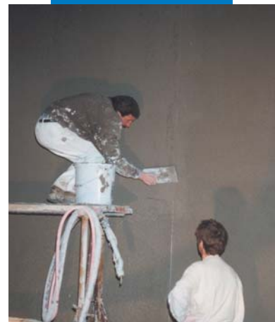
Smoothing with a float
